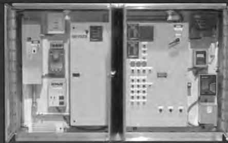
Pad Mounted Control Packages
